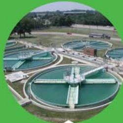
Sewage Treatment Plants
